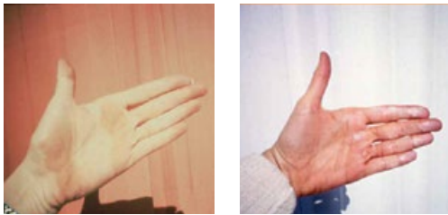
Failure in the Resin System Causes Chalking
